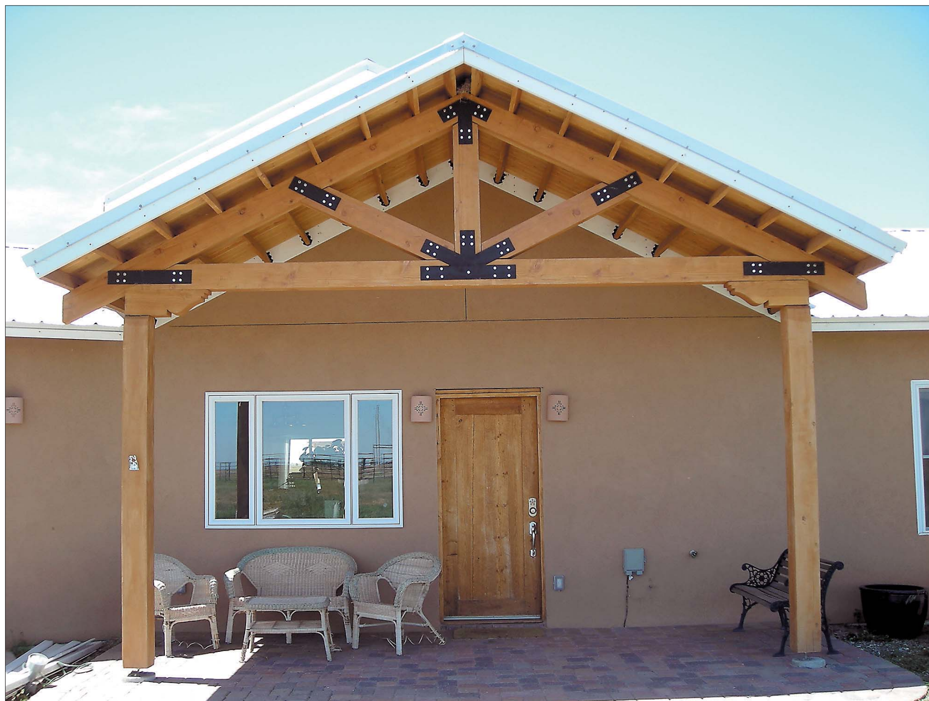
Project DIY helped homeowner Jack Bermudez consider all the options for a porch addition. The result you see above.
