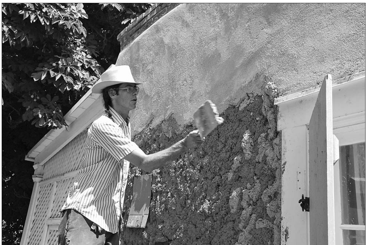
Ian Daitz, one of the workshop instructors, throws mud and works with lime plaster at El Zaguán on Canyon Road.
